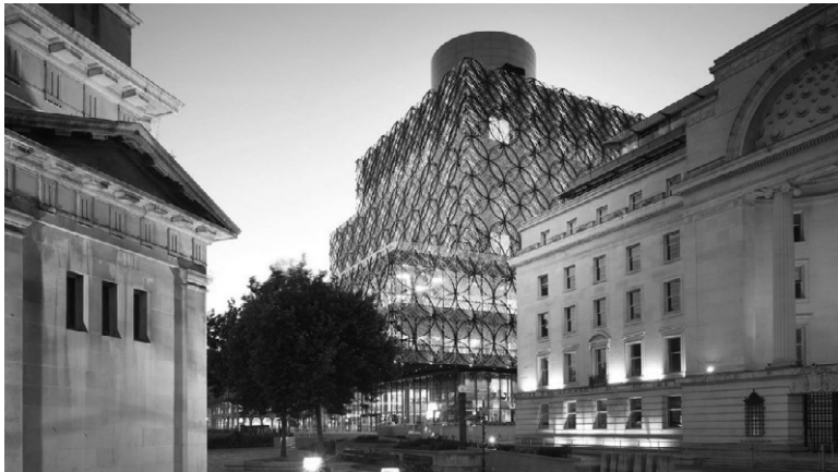
Fig. 2. The Library of Birmingham, UK (Source: Image provided by Mecanoo architects, Image copyright by Christian Richters)
